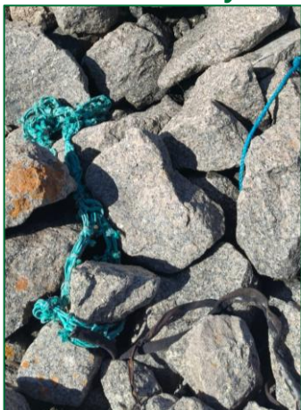
Figure 24. Green rope found along breakwater
