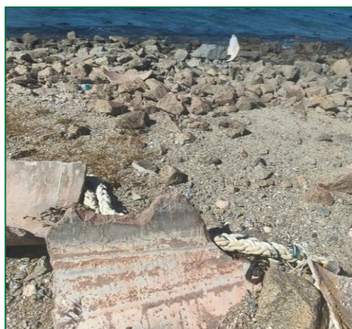
Figure 31. Large rope found along the breakwater
