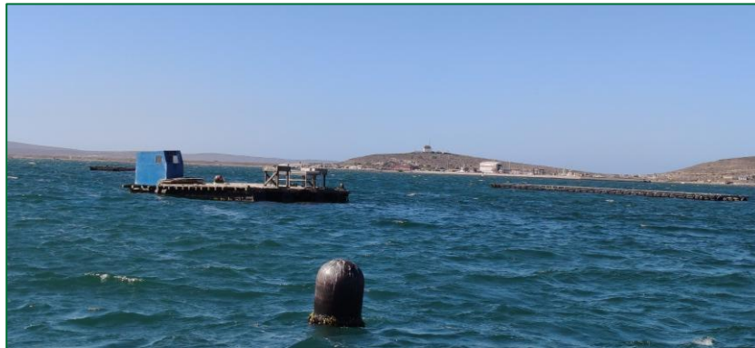
Figure 7. Service barge noted to be free of equipment and waste. No loose infrastructure observed.
