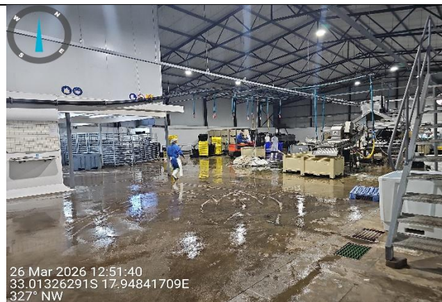
Photograph 83: Removal of the shells inside the processing factory of SBOC.
