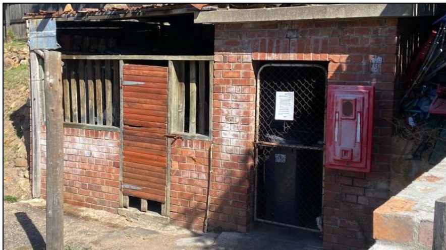
Figure 10. The dedicated waste storage area at Miller's Point Resort was all in order.
