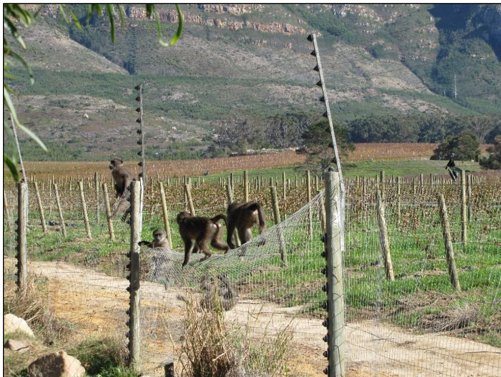
Figure 17. The fence at Buitenverwachting needs repair and is not currently baboon-proof.
